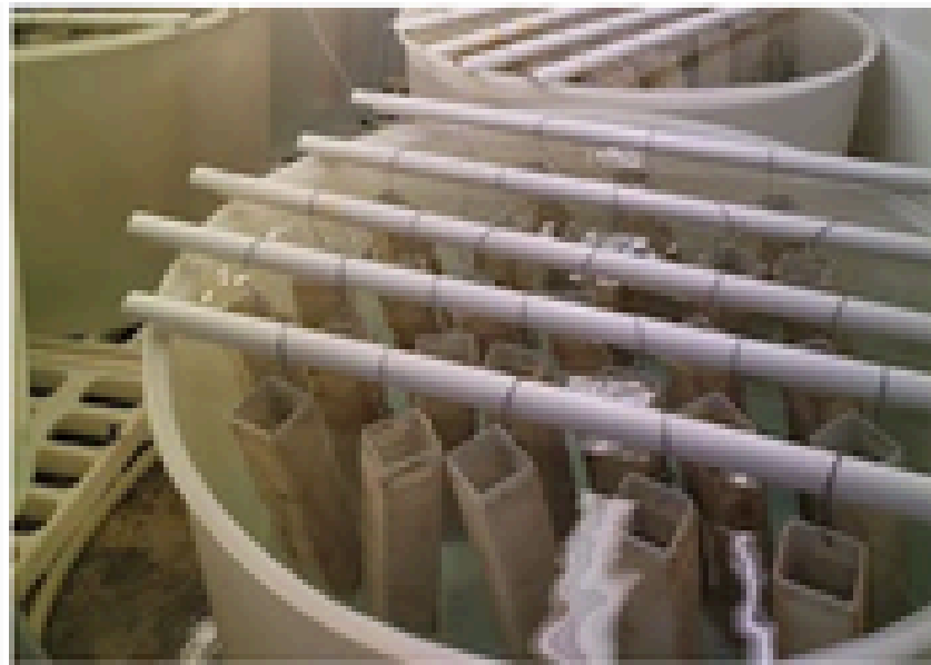
Seaweed Hatchery Facilities
